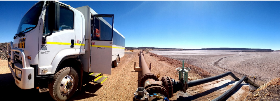
Tailing facility in the middle of nowhere
