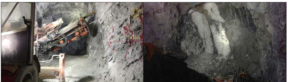
Figure 3: Jumbo twin boom drill
