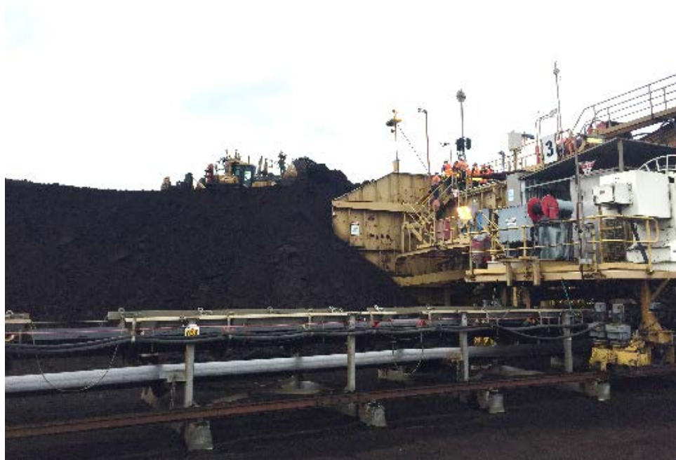
Figure 6: Dozer and Feeder Station, Photo by S. Leonhard
